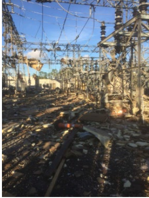
Fig. 10 Example of Storm Damage to AIS Structures Exposed to the Environment
