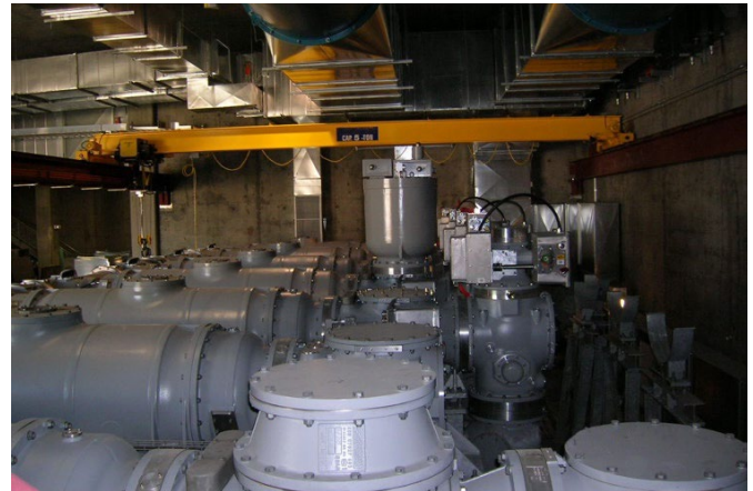
Fig. 13 Interior of Underground GIS
